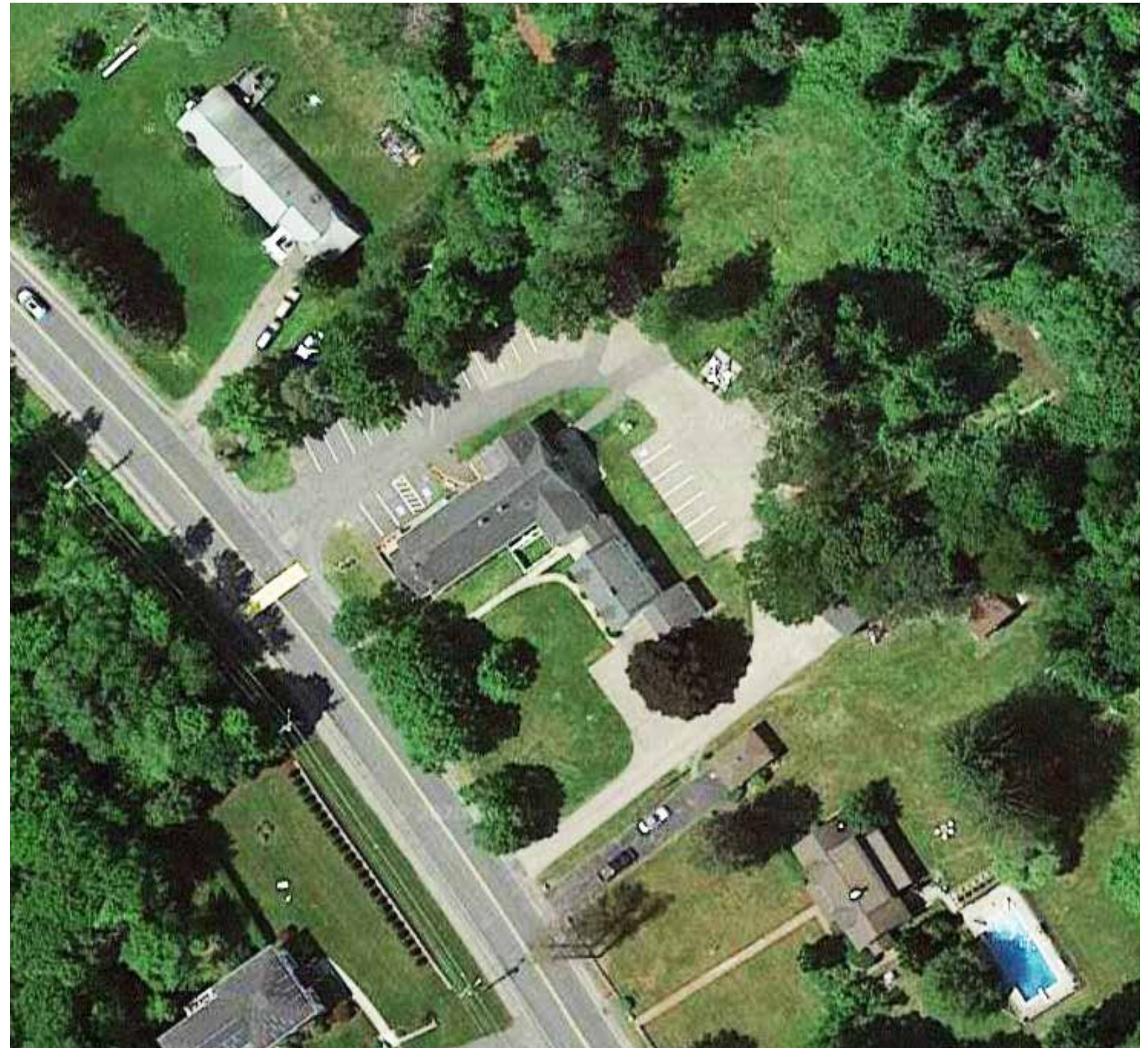
AERIAL VIEW OF EXISTING BUILDING AND SITE
